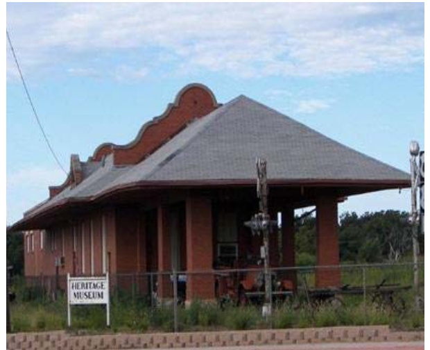
Quanah, Acme and Pacific Railroad Depot now our Heritage Museum.
